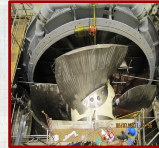
Webbers Falls Turbine
